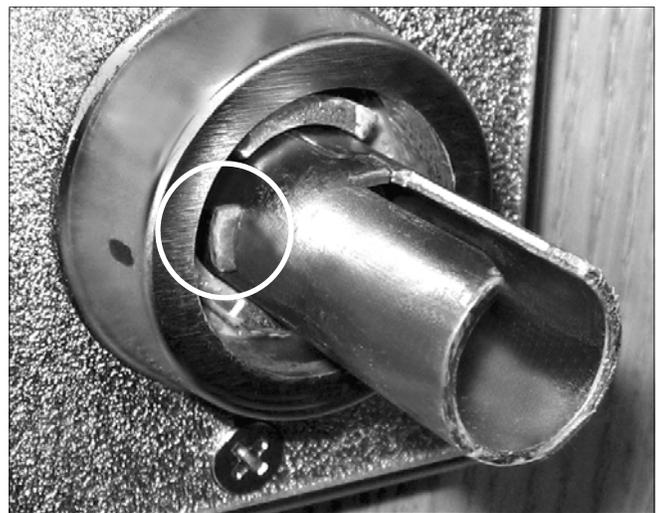
FIG. 6: PUSH IN LEVER CATCH (CIRCLED)
