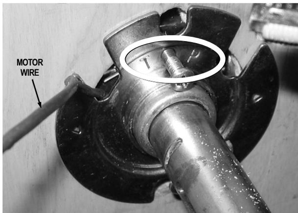
FIG. 12: INSIDE ROSE PLATE INSTALLATION
